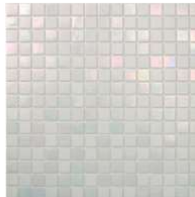
WF 4 shower recess finished in dj 7155 mosaic
